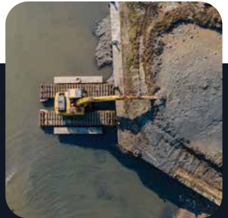
SHORELINE AND COASTAL MAINTENANCE
