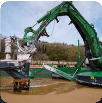
DREDGING AND UNDERWATER EXCAVATION
